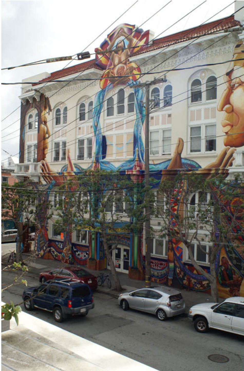
Photo 1. North (primary) façade, looking southeast.
