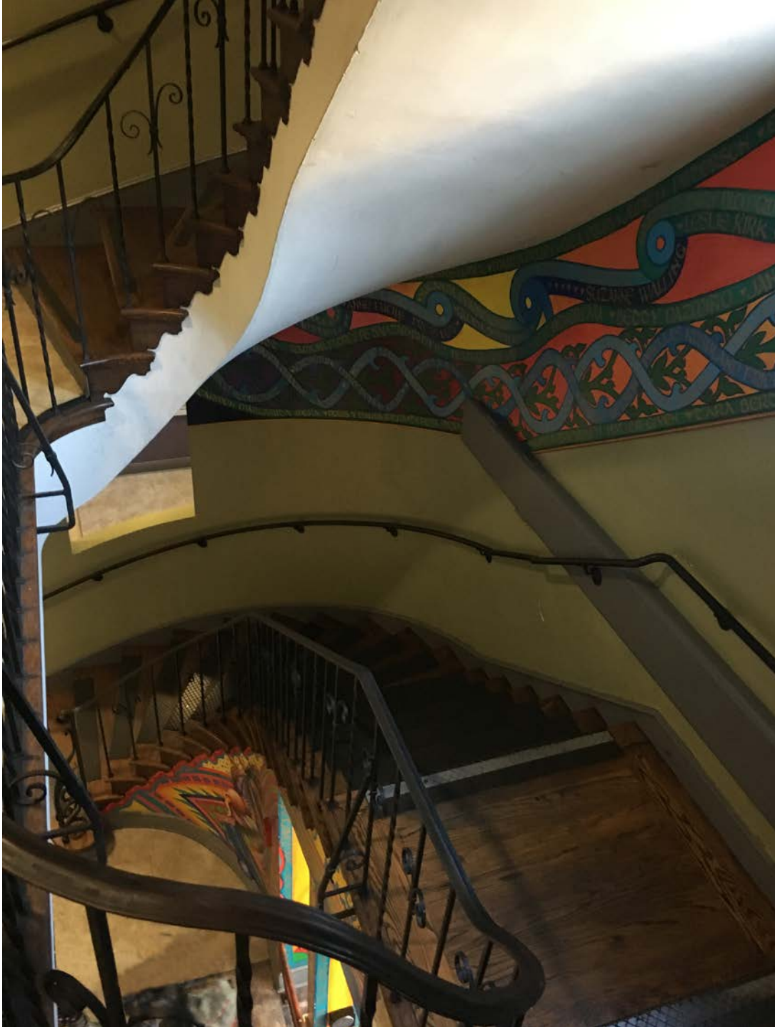
Photo 14. Second level interior, stairwell, looking down.
