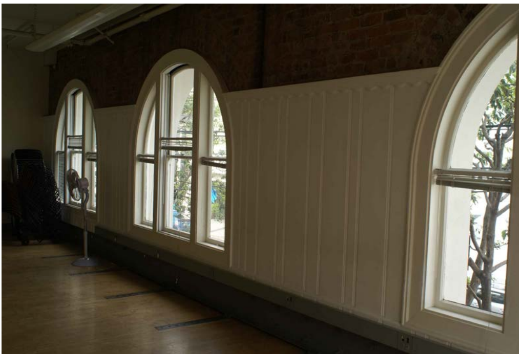
Photo 18. Second level interior, classroom detail, showing typical arched tripartite windows, beadboard, scalloped molding and exposed brick, looking northwest.
