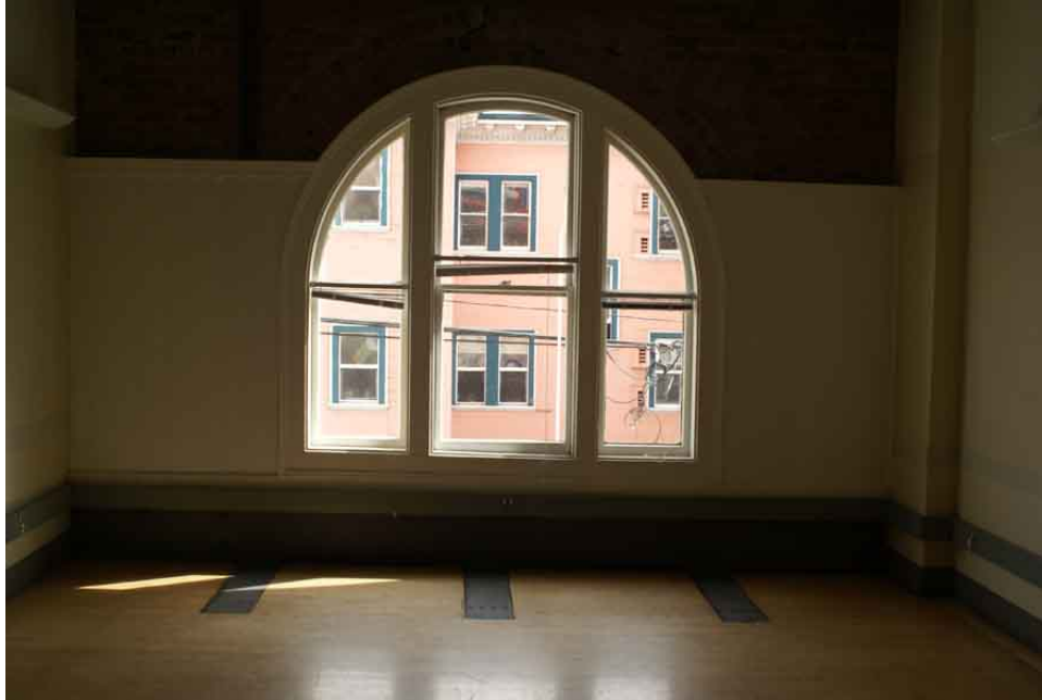
Photo 20. Second level interior, meeting room (Audre Lorde Room) showing typical arched tripartite windows, beadboard, scalloped molding, looking north.
