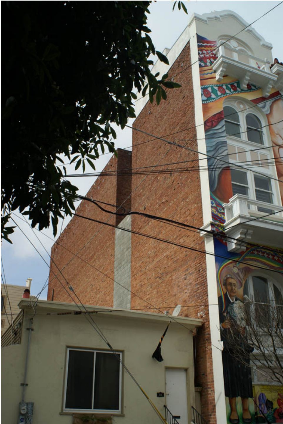
Photo 10. South façade, facing northwest.
