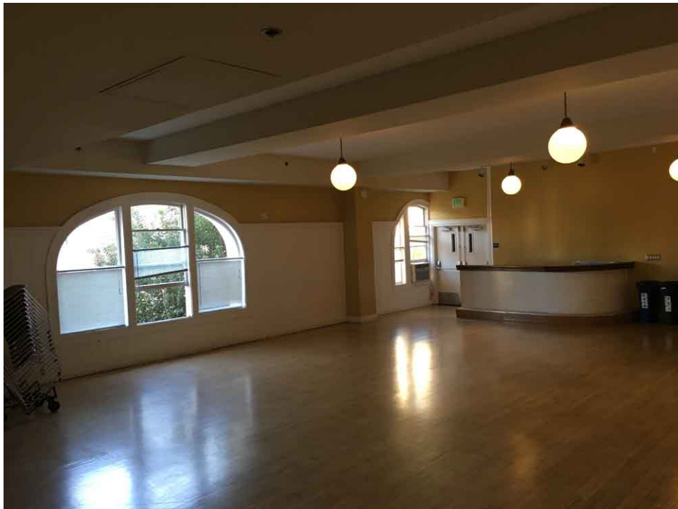
Photo 20. Second level interior, meeting room (Audre Lorde Room) showing typical arched tripartite windows, beadboard, scalloped molding, looking north.
